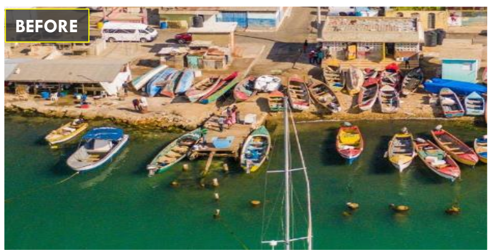
Old Ferry Pier Rehab
