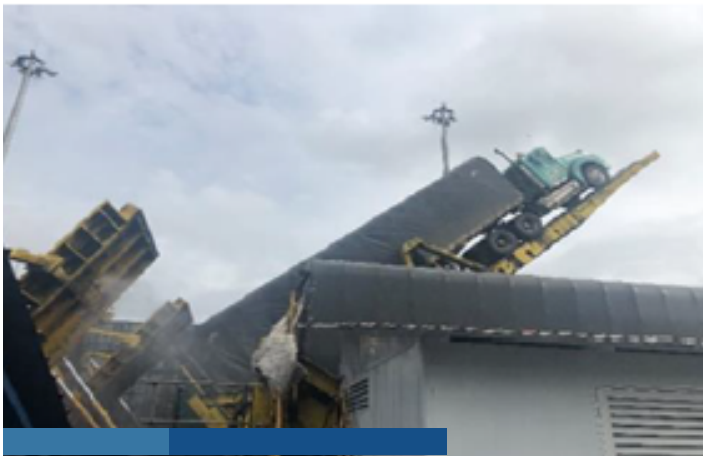
Dumpers with rainwater sprinkler system.
