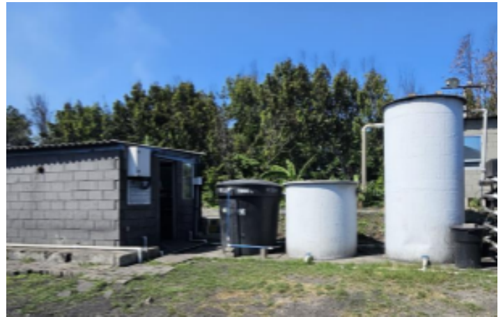
Side view of treatment plant, flocculation, filtration.
