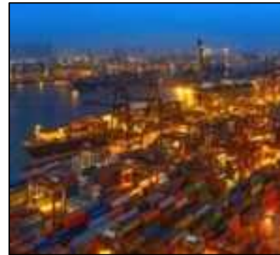
Ports & Terminal Operators
